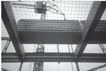
Figure 5.33: Left, prefabricated-removable floor elements placed on the first floor and 3D representation of theXX building structure (right)
