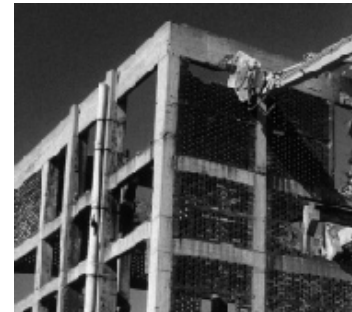
Figure 1.07: Demolition sequences of the concrete structures using breaker shears
