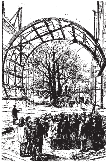
Figure 4.01: Assembly of one segment of the Crystal Palace in London by Joseph Paxton with Fox and Henderson Construction Engineers 1851
