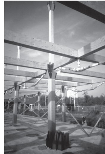
Figure 5.31: post and beam structure of the XX building
