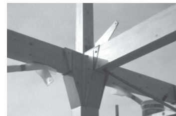
Figure 5.32: column – beam connection
