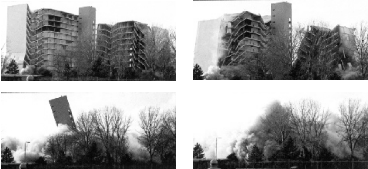
Figure 1.04: Demolition sequences with use of explosive
